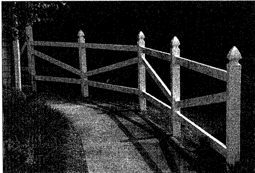
A newly installed section of vinyl fencing is featured in photo above.
